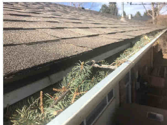
Winter winds can add a surprising amount of debris to the gutters.
